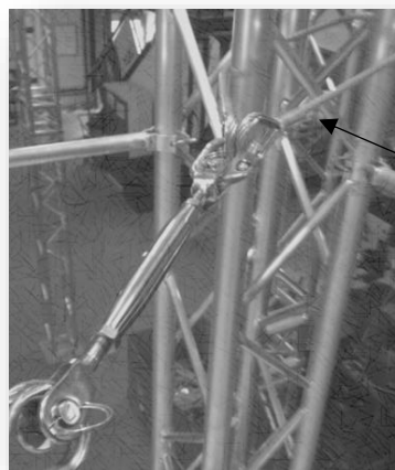
Picture 1 : Put sling around the anchorage
