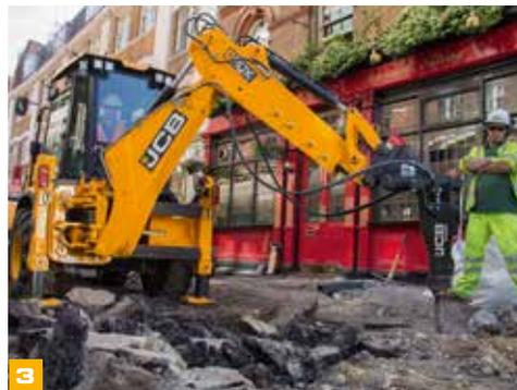
**4** Under 6m turning circle means it can work in a single carriageway allowing a road to be kept open.
