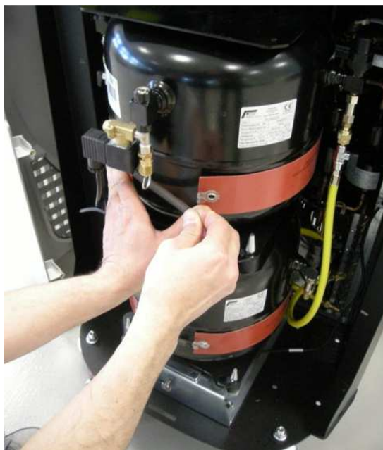
Image 4.64 – Removal of the heating band from the upper tank of the Konfort 780R BiGas
