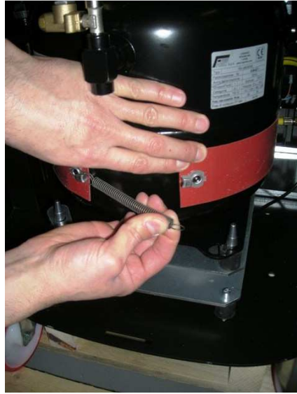
Image 4.21 – Heating band removal from the refrigerant tank
