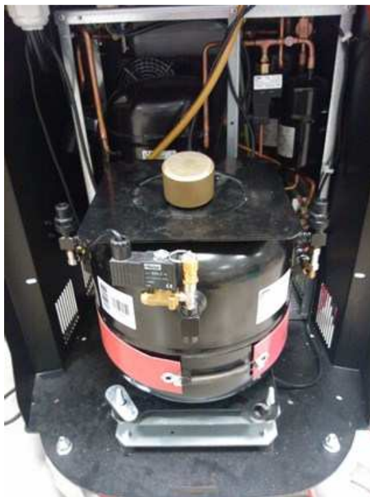
Image 4.30 – Placement of the sample weight on refrigerant tank
