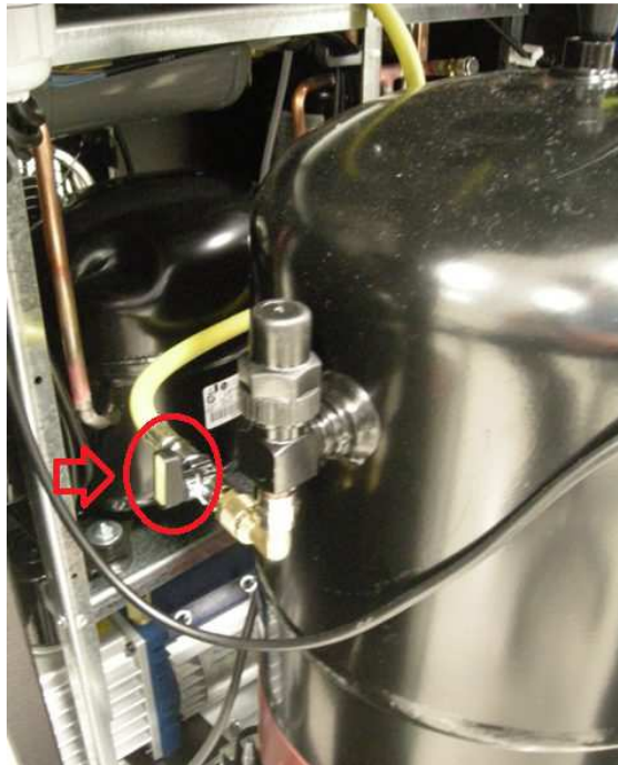
Image 7.25 – Closure of the outlet valve of the tank
